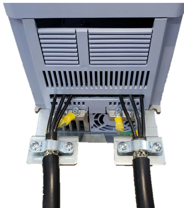
Figure 3.16: Detail of the motor cable shield connection
