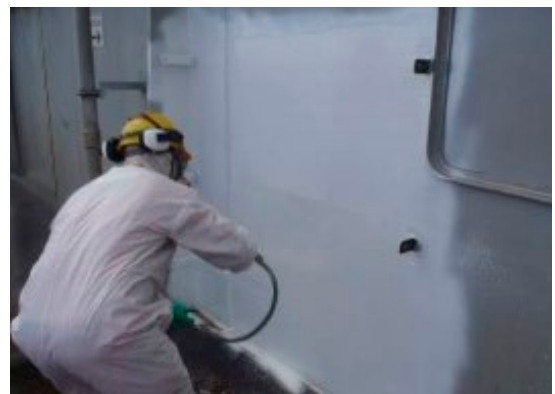
Apply over hydroblasted surfaces in grade CWJ-2 according to SSPC-VIS 4 Standard.
