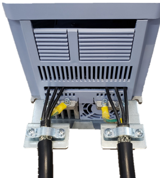
Figure 3.28: Detail of the power cable shield connection
