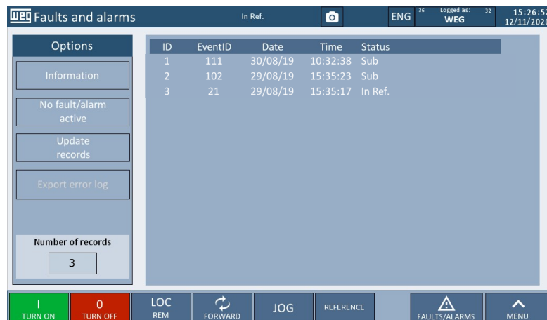
Figure 4.30: Fault and alarm history
