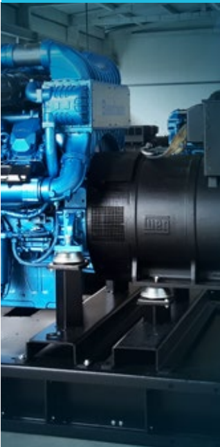
Distributed power generation 25,000 kVA
