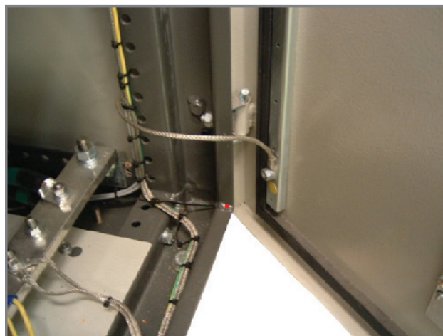
Figure 3.55: Grounding of the panel door
