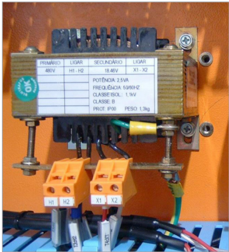
Figure 3.42: Mounting example of the transformers
