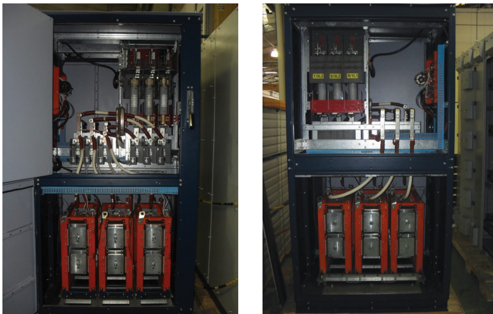
Figure 5.8: Medium voltage compartment (from view and rear view) – IP41
