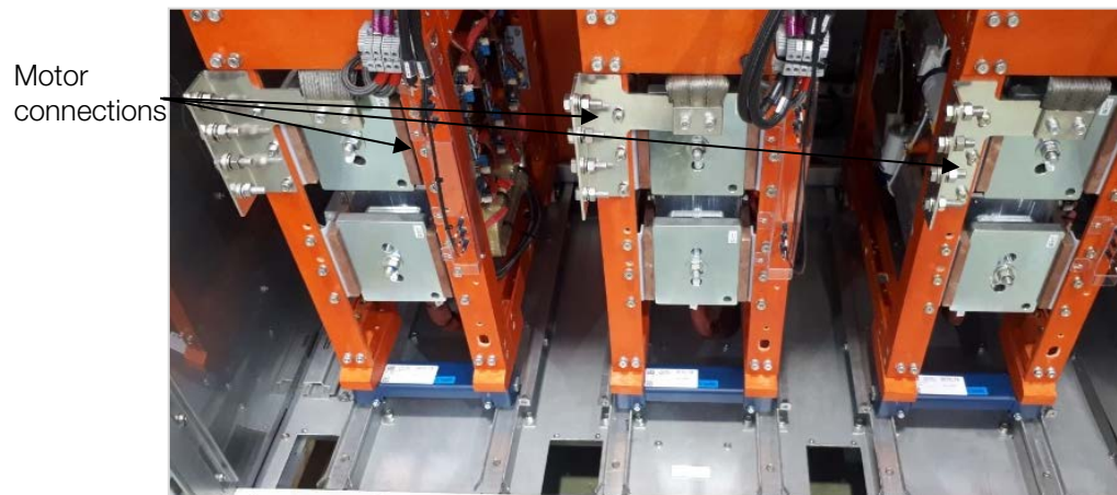
Figure 5.30 (c): Front panel view. Motor connections – SSW7000D IP41
