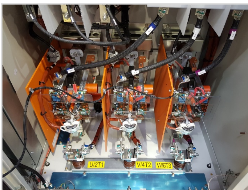
Figure 5.18 SSW7000C Power arms installation.
