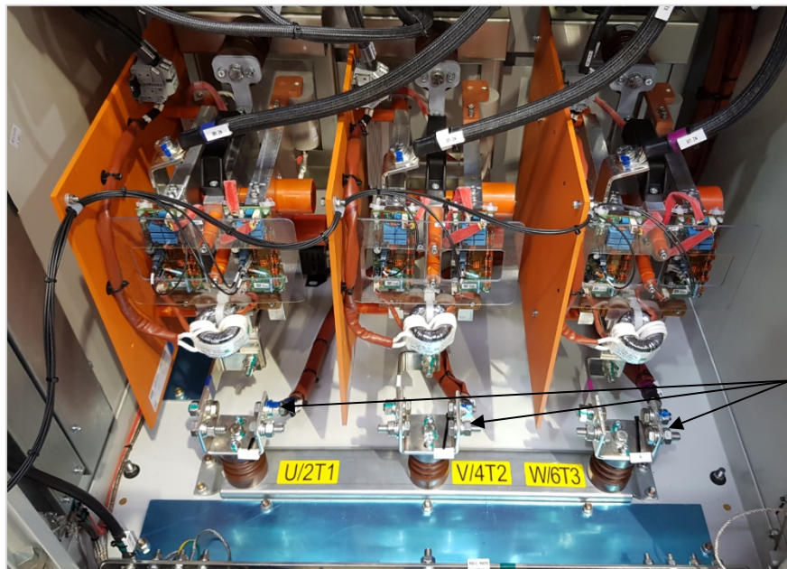
Figure 5.30 (b): Front panel view. Motor connections – SSW7000C
