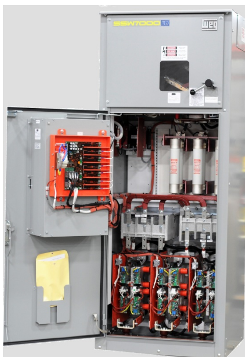
Figure 5.9: Medium voltage compartment (front view) SSW7000C – Nema 12
