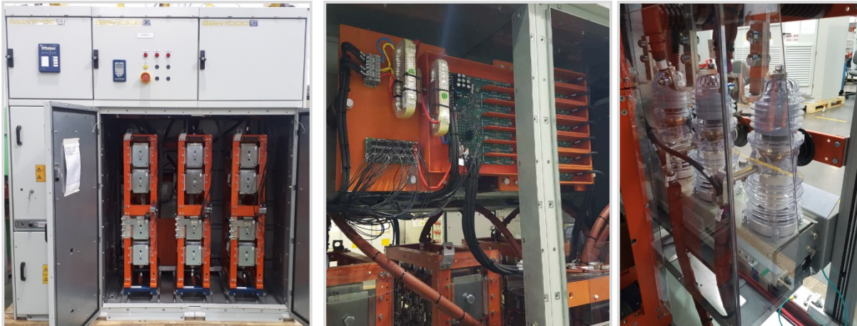
Figure 5.10: Medium voltage compartment (front view and back view) SSW7000D – IP41.
