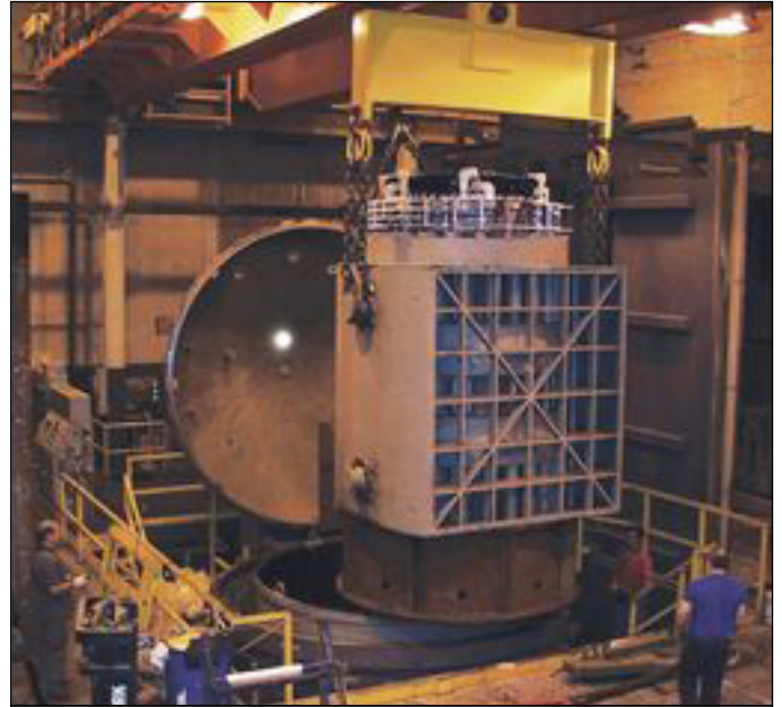
Wound stator entering the VPI tank for impregnation
