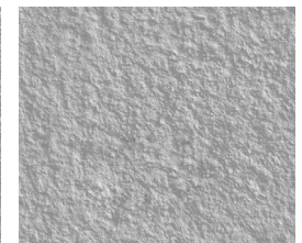
CSP 5 – medium shotblasting 1676,4 µm*
