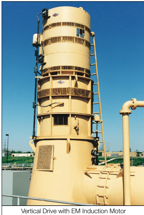
Vertical Drive with EM Induction Motor
