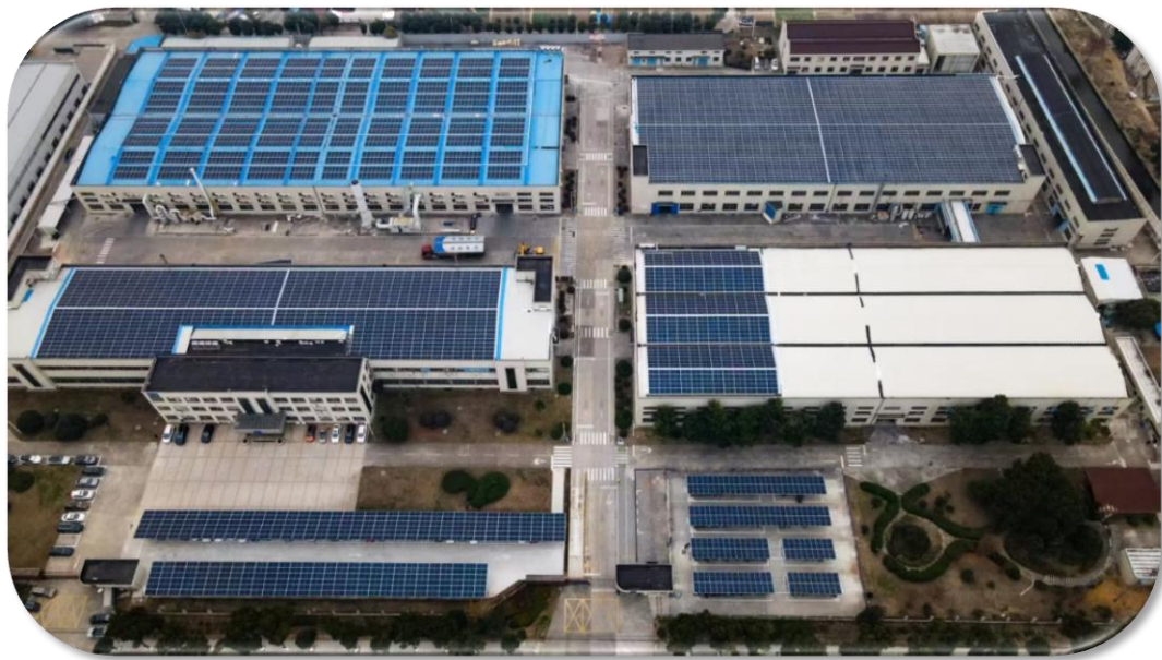
Solar panels installed on the WCZ rooftops
