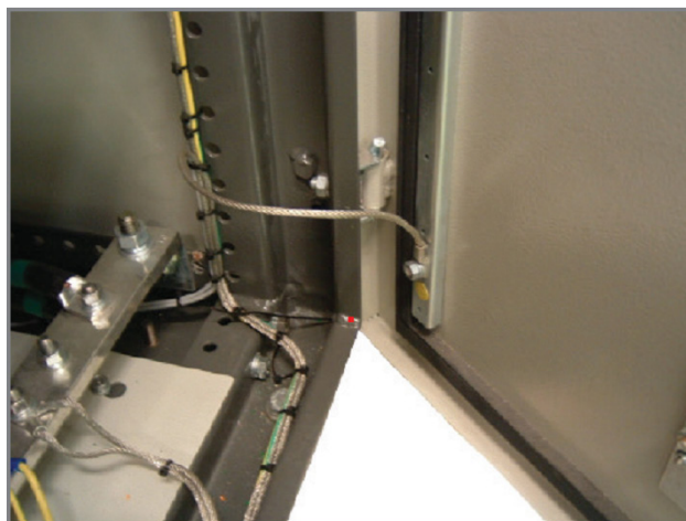
Figure 3.39: Grounding of the panel door
