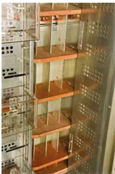
Vertical busbar protected by metallic cover, with openings to allow thermal camera inspection
