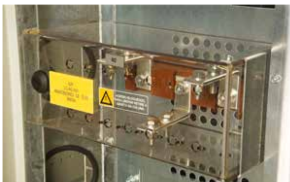
Individual plexiglas protection covers, with openings to allow thermal camera inspection
