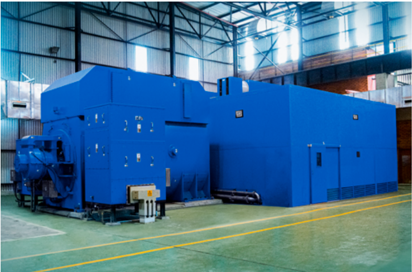
Higher level installation with civil base, downward radial exhaust and 2-pole generator.
