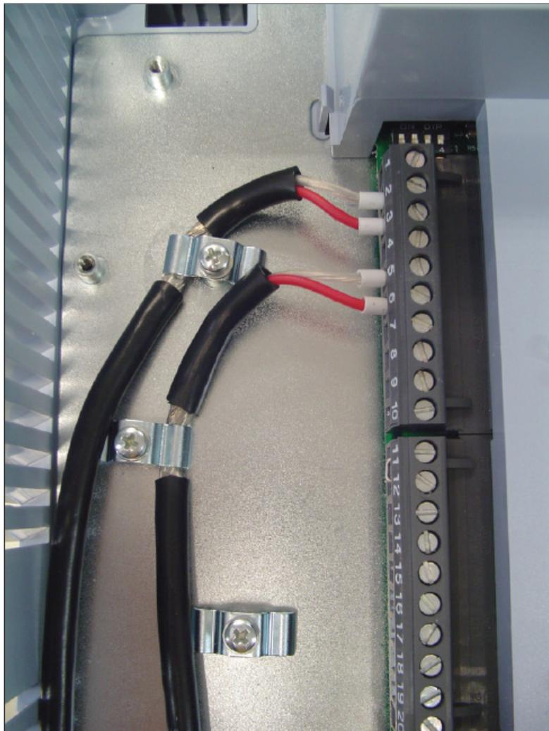
**Figure 3.43:** Example of shield connection for the control wiring
