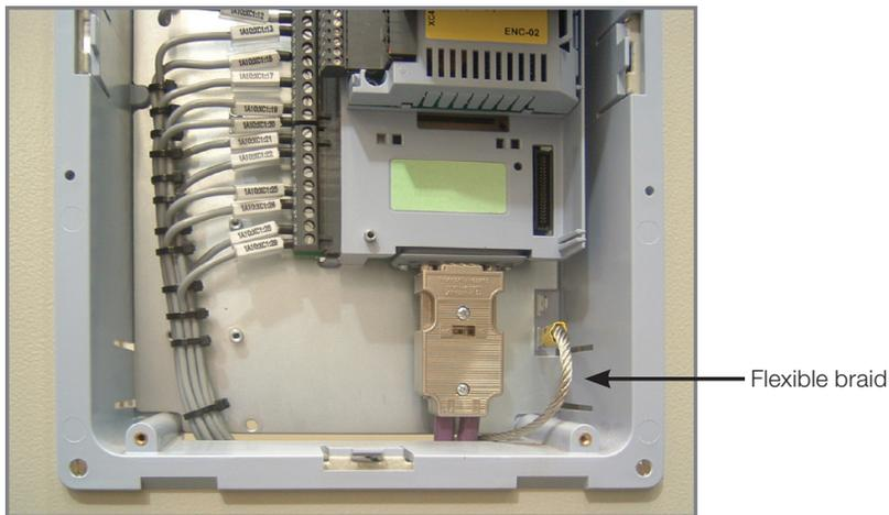
Figure 3.37: Control rack grounding
