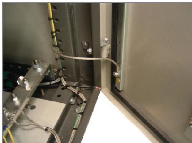
Figure 3.38: Panel door grounding
