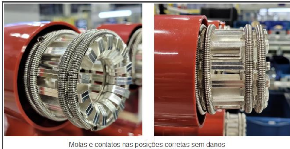
Figure 9.2: Circuit breaker springs and contacts
