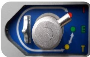
**INSERTED Position (I):** Power and control stabs are connected and the unit is ready for operation. The change to TESTING position is not permitted without first turning the functional unit off
