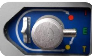
**EXTRACTED Position (E):** Power and control stabs are totally disconnected. In this position the total extraction of the functional unit from its compartment is possible and completely safe for the user
