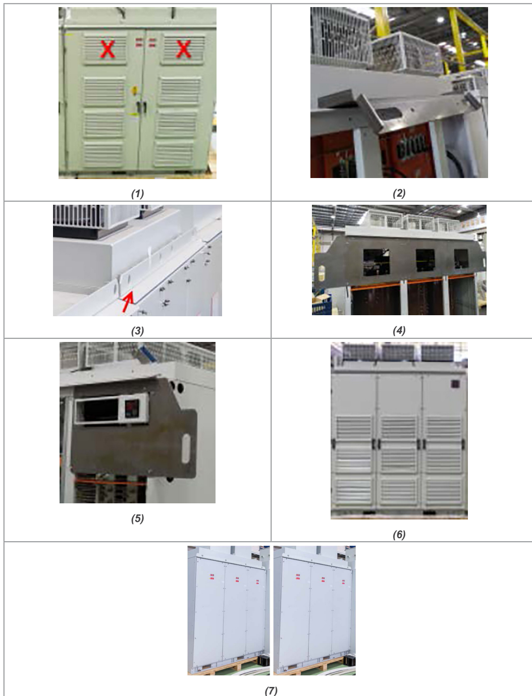
Figure 6.4: Procedure to remove the air transport reinforcements from the MVW3000
