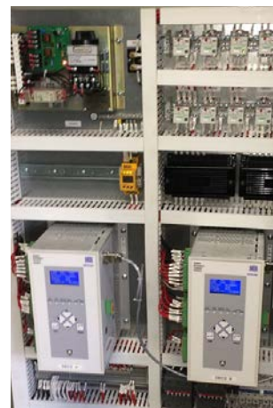
Redundant generator excitation and ground-detection system installed in major refinery
