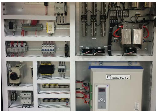
200-Amp digital excitation system for static motor or generator
