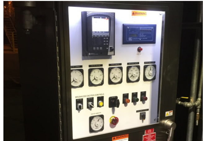
Complete motor excitation and protection cabinet suitable for Class 1, Div II areas
