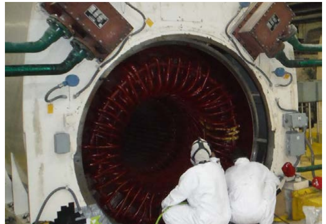
Painting and varnish treatment to OEM specifications
